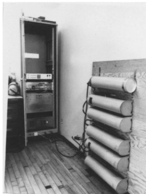
Cavities for the 2 meter repeater.
